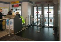
This record FlipFlow WIDE extended is installed at Glasgow International Airport. The units can be operated singly and so not used when not needed. The FlipFlow system allows safe and secure passage of persons into or from areas where security is a priority and a controlled flow of people is required.
