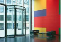
The east entrance at Tower Place in london was designed by architects Foster and Partners. This installtion is a fully automatic **record K41** four wing revolving door and has an all-glass drum with visible parts anodised. The operating drive for this revolving door is concealed beneath the floor in a casing which protects it from water and dirt.
